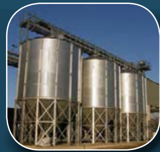
Hopper Bottom Silos
