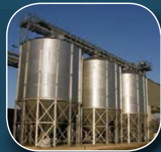
Hopper Bottom Silos
