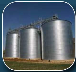
Flat Bottom Silos
